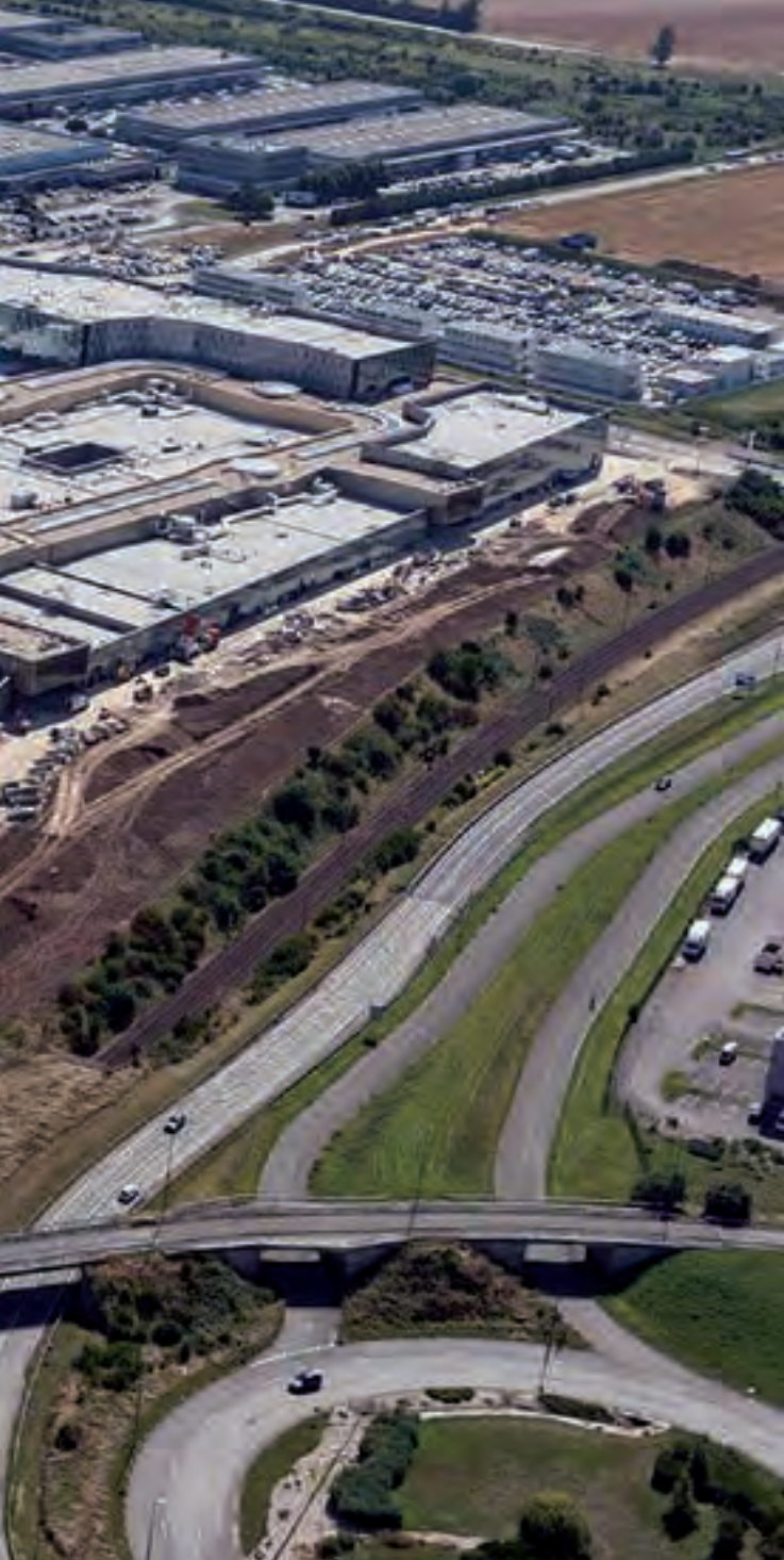
Aerial view of the site Vista aerea del cantiere
